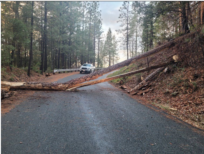
Figure 7. A tree blocking the road at Paradise Lake.
