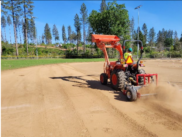
Figure 7. Reconditioning the infield of the small ball field.
