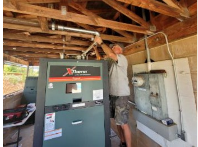
Figure 4. New boiler being installed at the pool.
