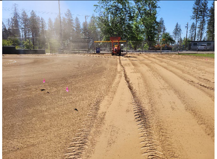
Figure 6. Reconditioning the infield of the small ball field.
