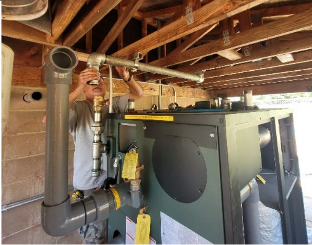
Figure 3. New boiler being installed at the pool.
