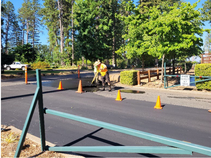
Figure 1. Maintenance workers laying new asphalt sealer.
