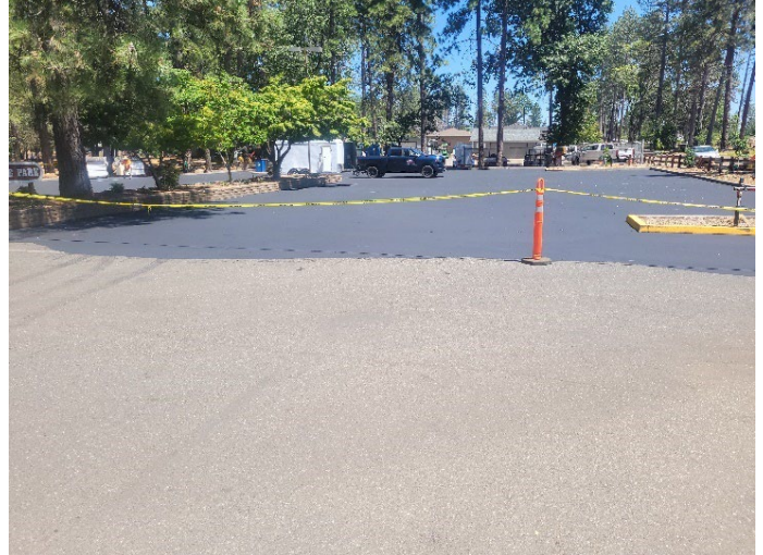
Figure 2. Lower Bille Park parking lot before new paint.
