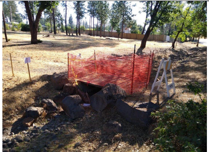
Figure 4. The old makeshift bridge at Bille Park.
