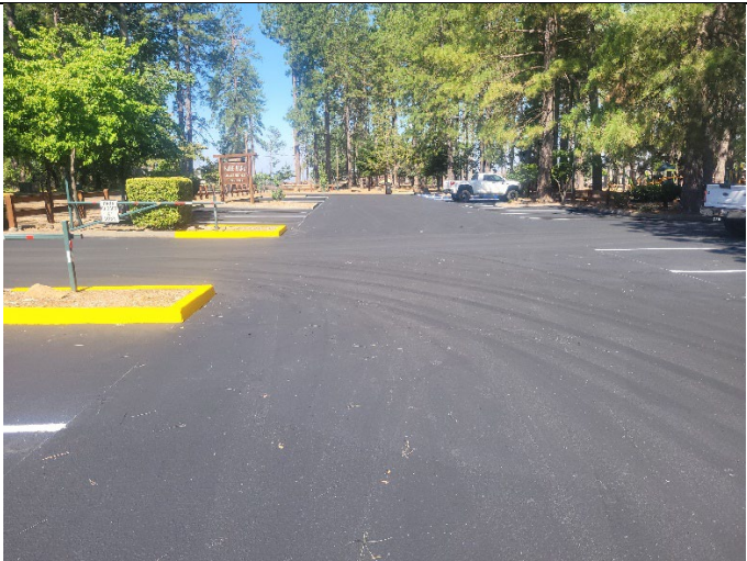
Figure 3. Upper Bille Park parking lot after being repainted.
