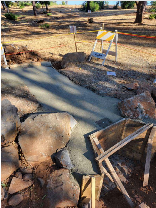
Figure 7. Cement drying for the completion of the walking bridge.
