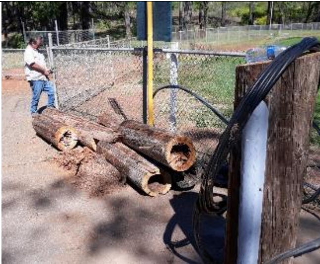
Figure 7. Hazard poles on the ground
