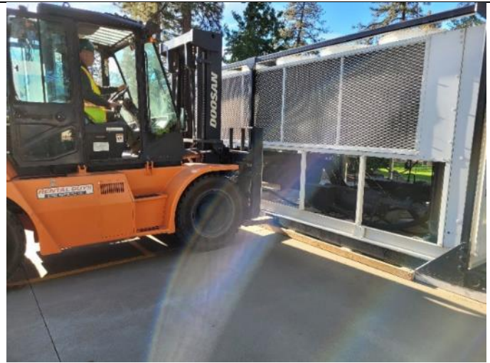
Figure 10. Chiller getting put into place for the Ice Rink.
