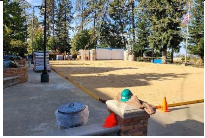
Figure 14. The Ice Rink being staged for set up.
