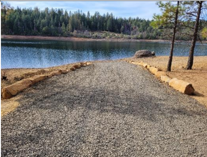
Figure 9. Newly improved and finished boat ramp.
