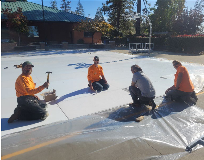
Figure 3. Maintenance putting together the Glice floor pieces.
