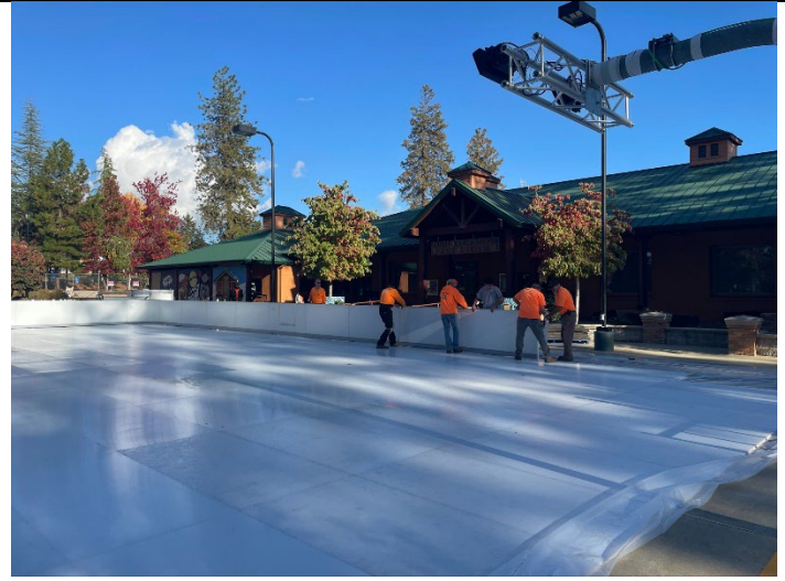
Figure 4. Maintenance putting up the walls to the Glice rink.
