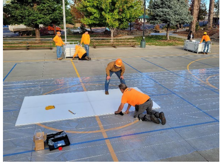
Figure 2. Maintenance putting together the Glice floor pieces.
