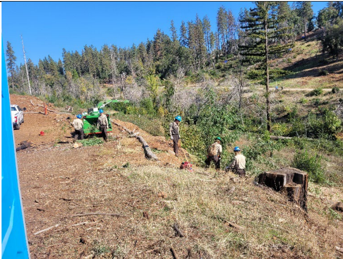
Figure 7. CCC Crew clearing our brush at Oak Creek Park.
