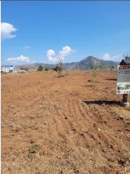
Figure 5. Cleared brush at the Lakeridge Park site.
