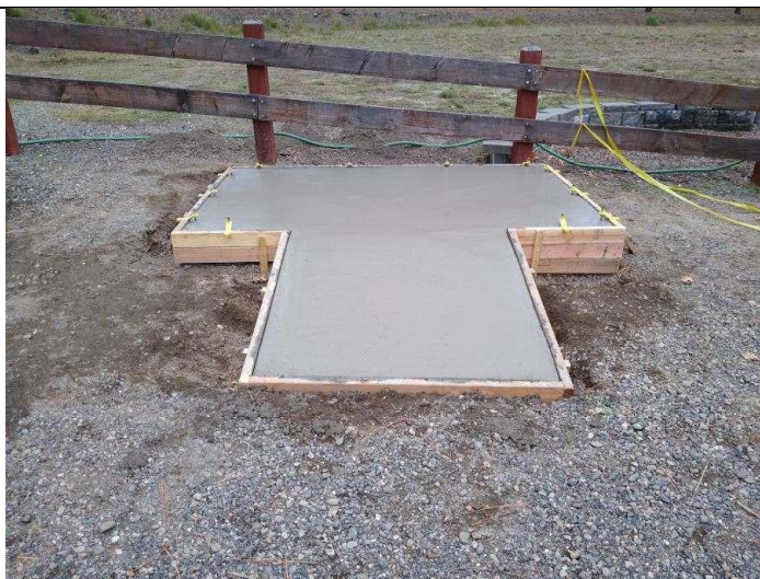
Figure 4. Trash bin storage pad.
