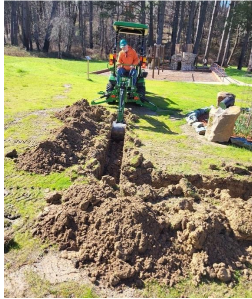
Figure 2. Ray Lockridge digging a trench for the new irrigation at Crain.
