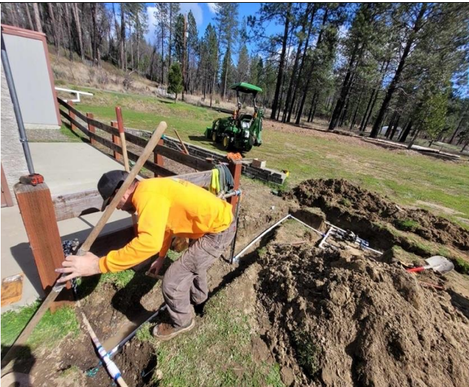
Figure 3. New irrigation pipes being put in.
