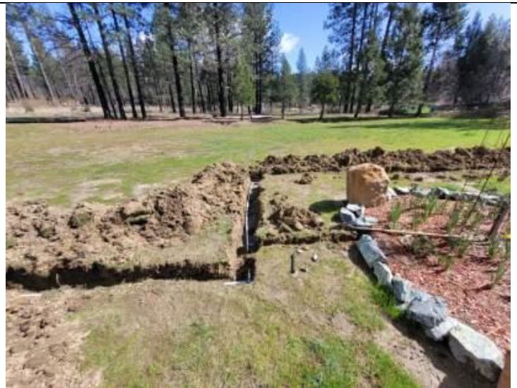
Figure 4. New irrigation at Crain Park is completed.
