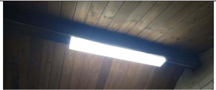
Figure 10. Lights after being replaced at Bille Park.
