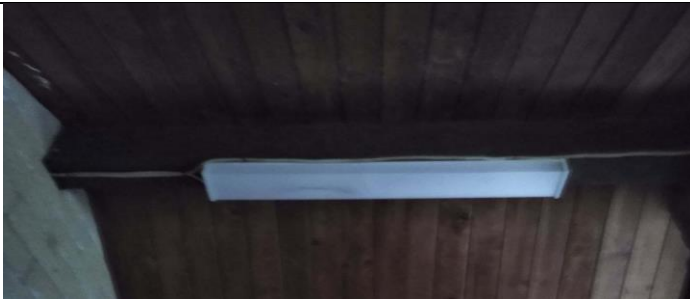
Figure 9. After the recent storm there were several lights that needed fixing.
