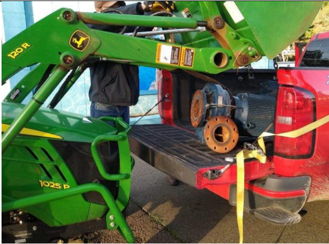
Figure 7. Park Maintenance using a tractor to lift the pool pump.
