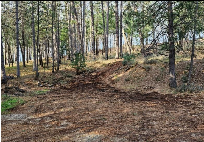
Figure 17. After all the logs were cleared.
