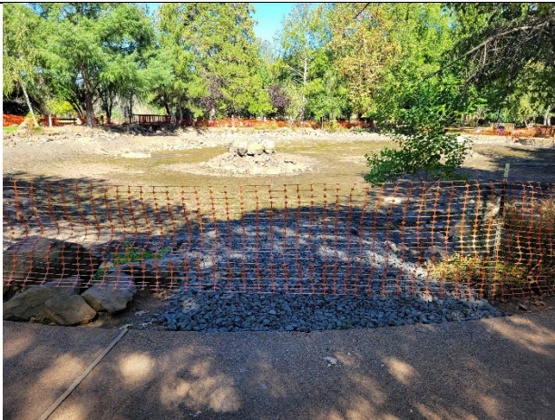
Figure 3. Finalizing the drain of the Aquatic Pond.
