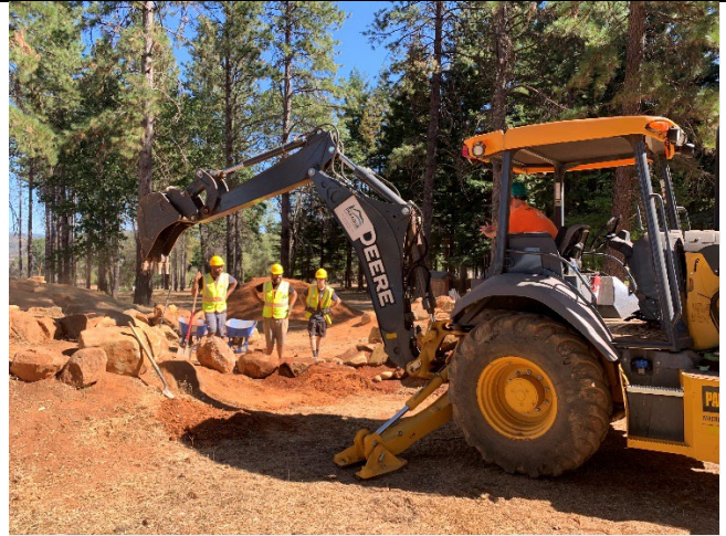
Figure 14. Before photo of new added feature - AMAIN volunteers directing tractor on rock layout.
