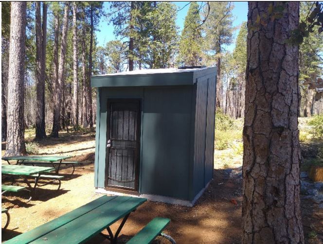
Figure 9. The pump house at Camp Coutolenc is finished.
