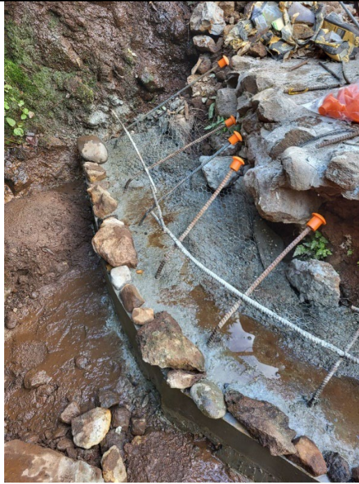
Figure 8. PRPD maintenance staff working on the rebuild of the grotto bridge.
