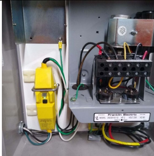
Figure 12. The replaced aerator at the Aquatic Park
