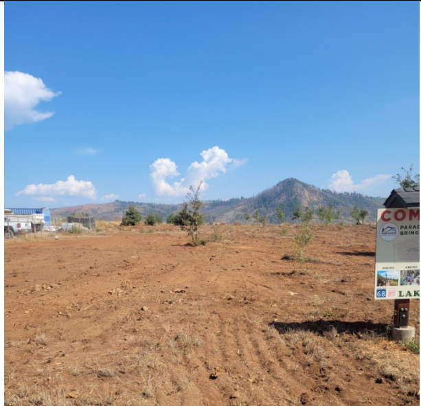
Figure 4. The Lakeridge Park site after the rough grading.
