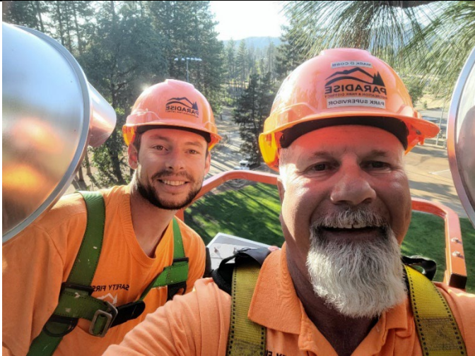
Figure 9. Mark Cobb and Spencer Strauss up high working on the lights at the ballpark.
