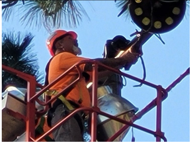
Figure 10. Mark Cobb replacing the broken light at the ballpark.
