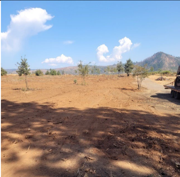
Figure 3. The Lakeridge Park site after the rough grading.
