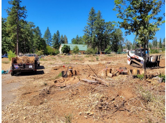
Figure 2. PRPD maintenance staff during the clearing and grubbing at the Lakeridge Park site.
