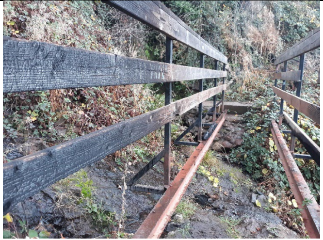
Figure 6. The bridge to the grotto prior to rebuilding.
