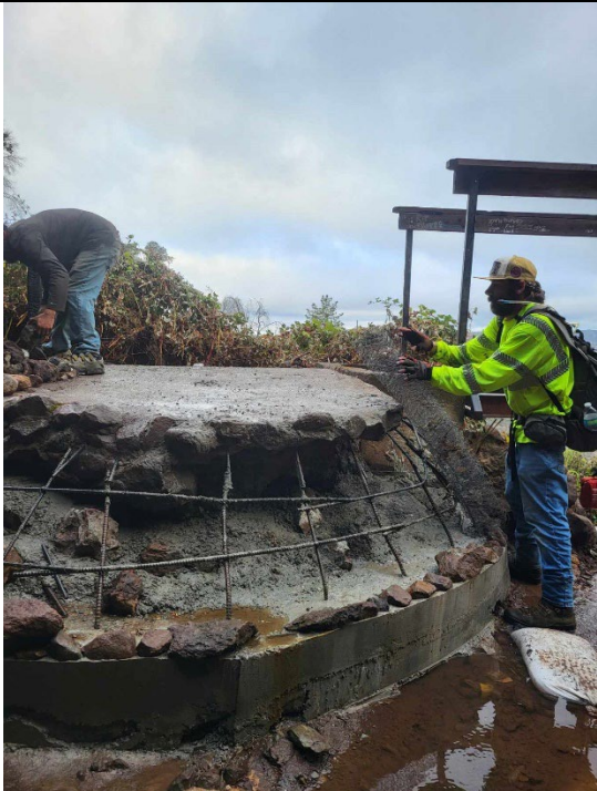
Figure 7. PRPD maintenance staff working on the rebuild of the grotto bridge.
