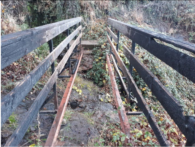
Figure 5. The bridge to the grotto prior to rebuilding.
