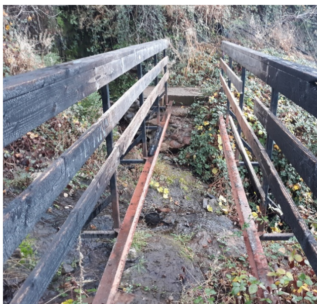
Figure 5. Grotto Bridge at Bille Park
