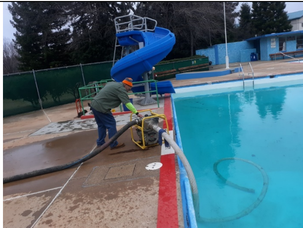
Figure 2. Pumping of pool begins (2/3/21).
