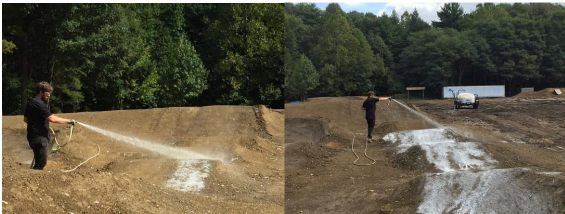
Applying soil stabilizer at the beginning of the season to extended the functional of a pump track.
