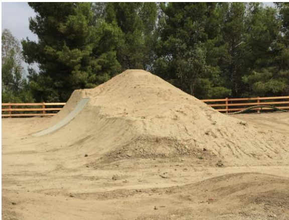
Final shape jump set with kicker lip on the front end and a lander transition on the back end.
