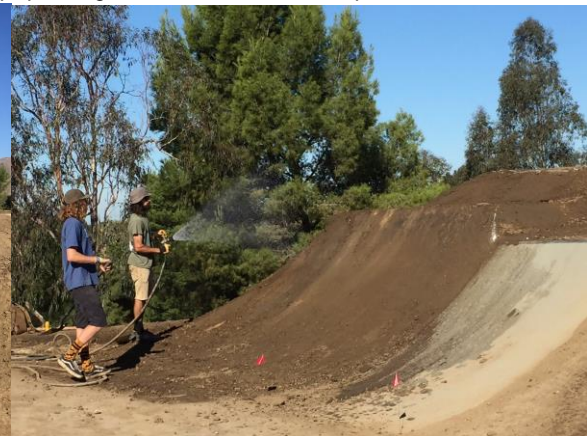
Continue to moisture condition, soil condition, shape and compact throughout the process.
