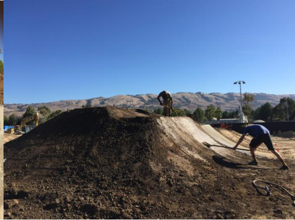
Using shovels to pack and shape dirt jump lip. Using the concrete kicker to shape to.
