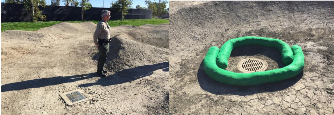
Winterizing drainage inlets with straw waddles and filter fabric will ensure they don't clog or release sediment into the storm water system.
