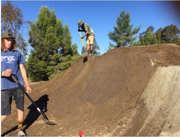
Using shovels to pack and shape dirt jump lip. Using the concrete kicker to shape to.
