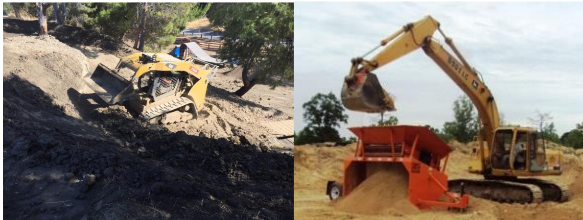
Conditioning a larger work area with a skid steer. Conditioning a soil stockpile with an auto sifter.
