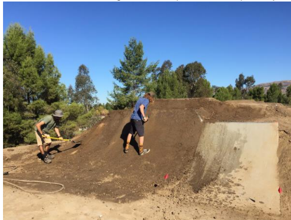
Continue to moisture condition, soil condition, shape and compact throughout the process.
