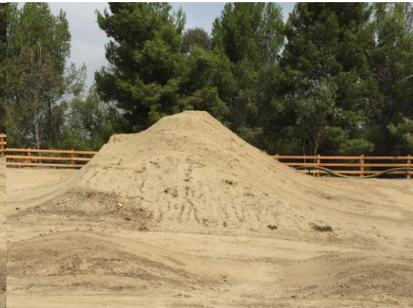
Final shape jump set with kicker lip on the front end and a lander transition on the back end.
