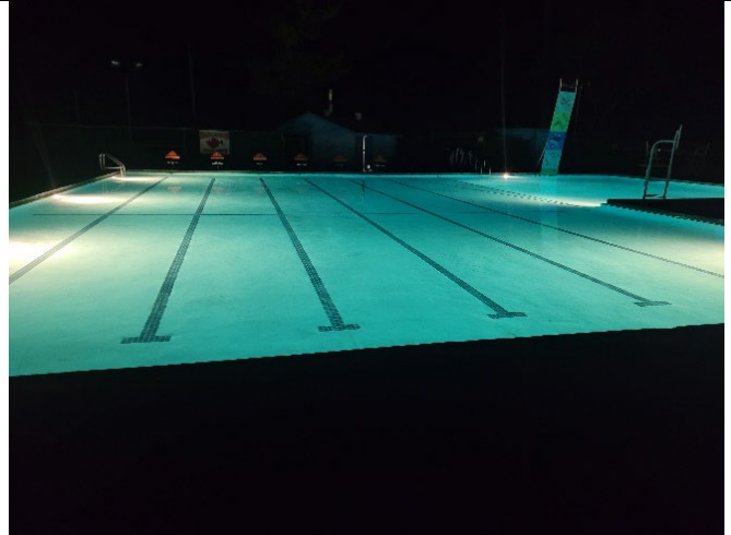
Figure 3. The new lights in the pool are working great and ready for the upcoming pool season.
