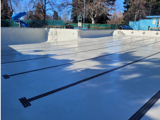
Figure 2. The pool with its new lining and tile work.
