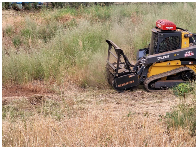
Figure 4. Clearing at the new shop property (before).
