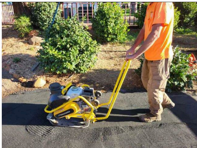
Figure 10. Maintenance workers laying gravel at the new Pollinator Garden.
