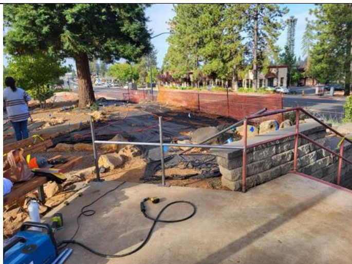
Figure 14. Railing is also going up around the Pollinator Garden.
