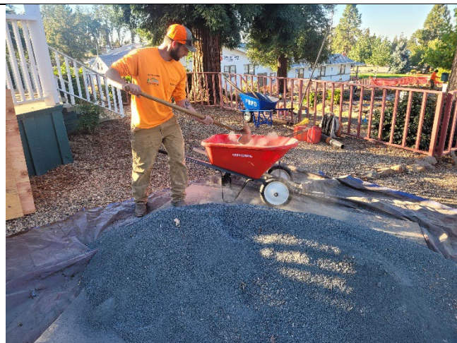
Figure 9. Maintenance workers laying gravel at the new Pollinator Garden.
