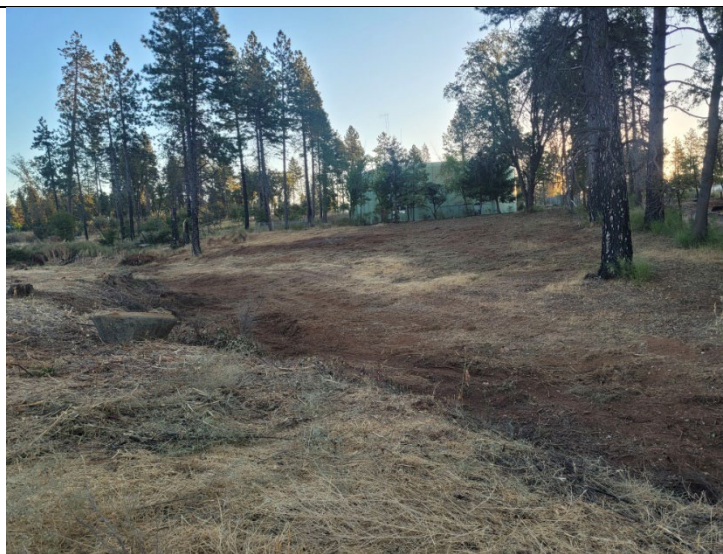
Figure 5. Clearing at the new shop property (after).
