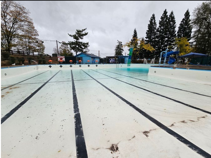
Figure 5. The pool in the process of being drained for relining.
